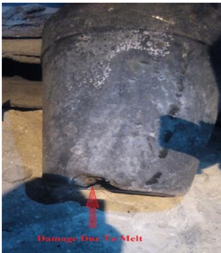
Figure 18. Newly developed tuyere with AM coating after damage and removal from the blast furnace
