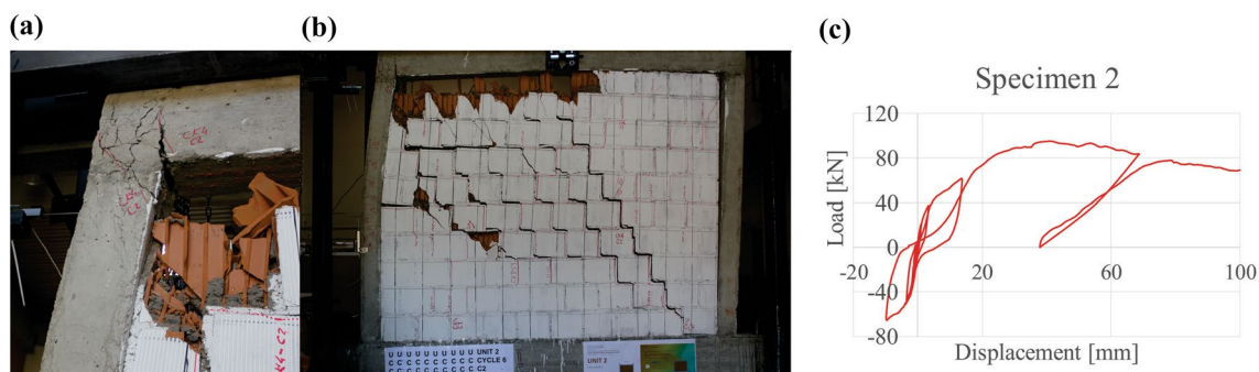
Fig. 7 Specimen 2, a details of the beam-to-column joints, b cracking of specimen 2 after test, and c lateral force–displacement response, Dautaj et al. (2018)
