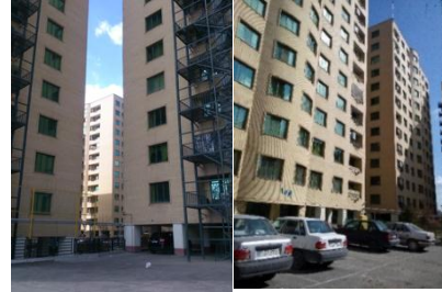
Fig. 4 . Blocks of Elahieh residential complex
