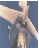
Fig. 1. The icing phenomena of a wind turbine.
