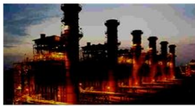
Combustion and Power Generation(3)
